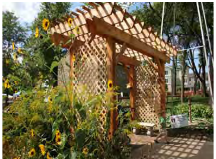
Completed pergola in Herb Garden at Legler Barn
